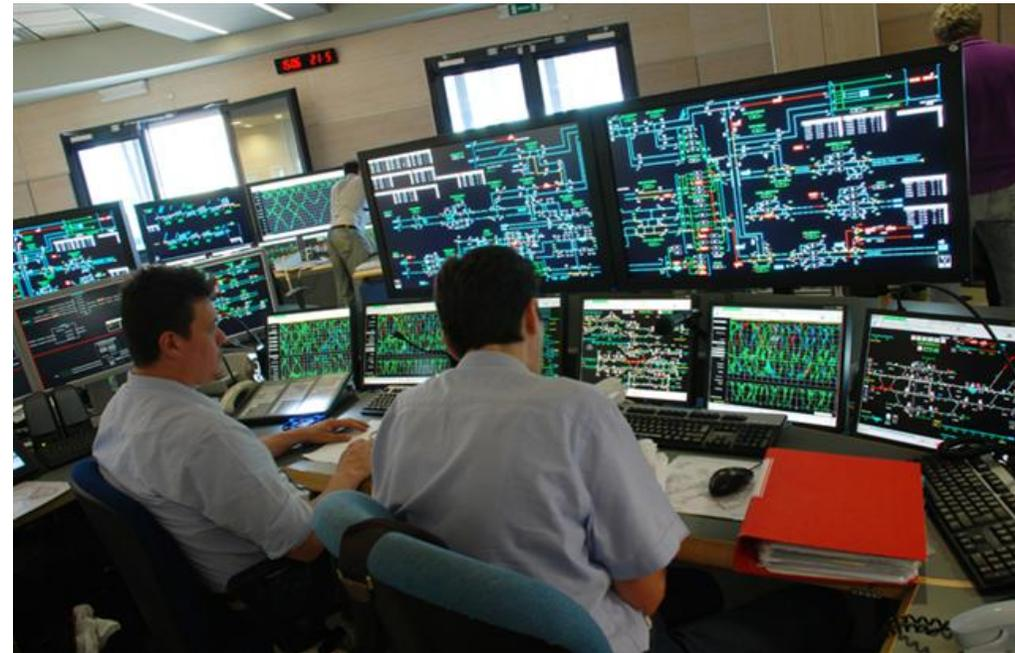
The Bologna Railway Node is the key junction between the North and the Centre of Italy's railway network. The Centralized Traffic Control controls 8 different lines, 78 stations or junctions and supervises the Bologna Centrale passing-through main station. An average of 1200 trains per day is managed by CTC.
